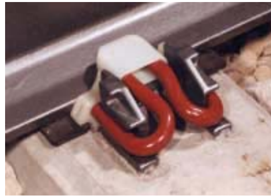
Figure 8.24: Pandrol Fastclip
