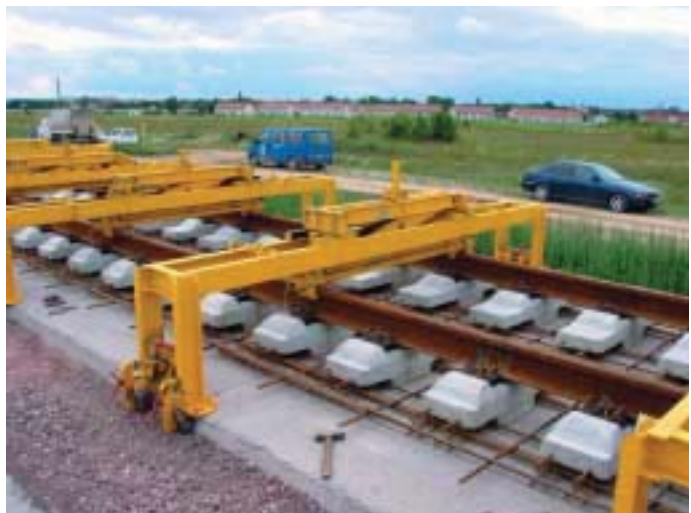
Figure 9.16: Alignment portals in the Leipzig-Gröbers project
