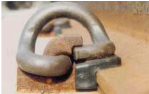
Figure 8.23: Pandrol fastening system
