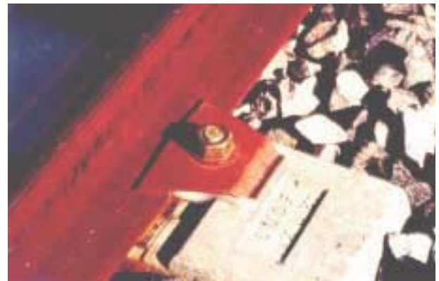
Figure 8.26: Nabla fastening system
