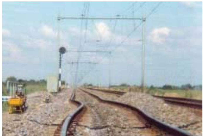
Figure 7.1: Example of track buckling
