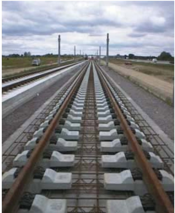
Figure 9.15: Track assembly, track on top of the concrete roadbed on the concrete roadbed (for the project Leipzig-Gröbers)
