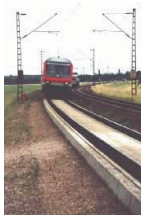
Figure 9.2: ... and slab track
